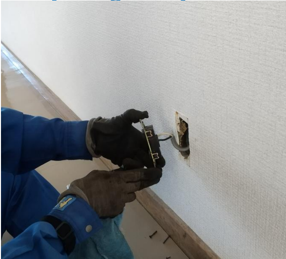
[Replacement of a defective outlet]
