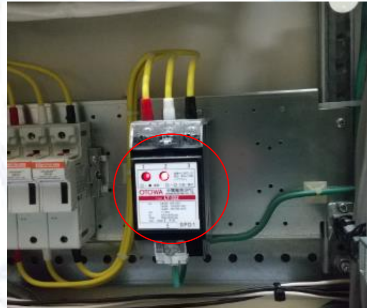
[Installation of a lightning arrester in a low voltage circuit]
