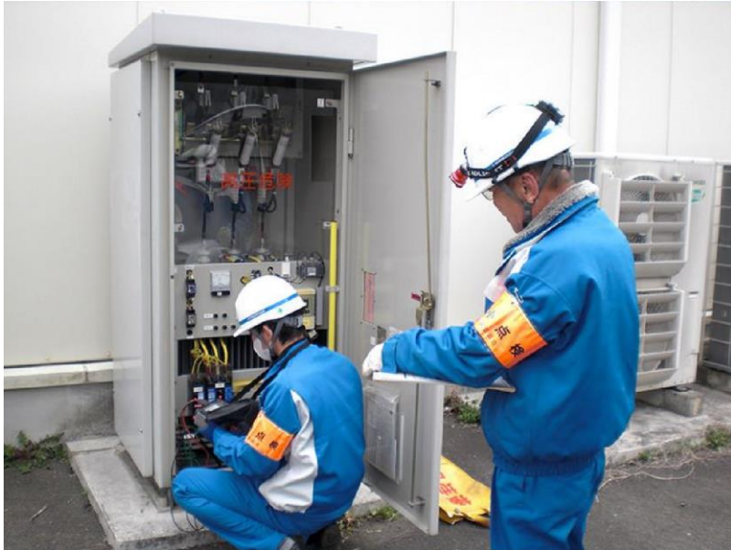
[Precision inspection by disconnecting demand equipment]
