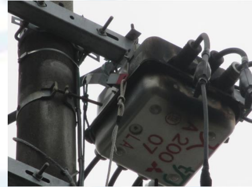
[Switchgear damaged by a lightning stroke]
