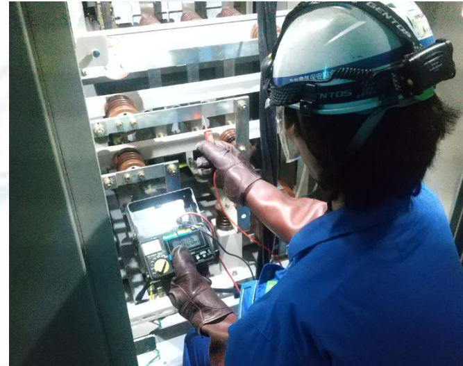
[Measurement of insulation resistance of electrical circuits]
