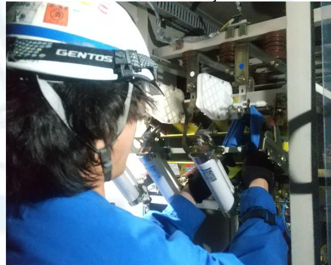
fisuel seminar – 15 and 16 October 2024 [Inspection and cleaning of electrical equipment]
