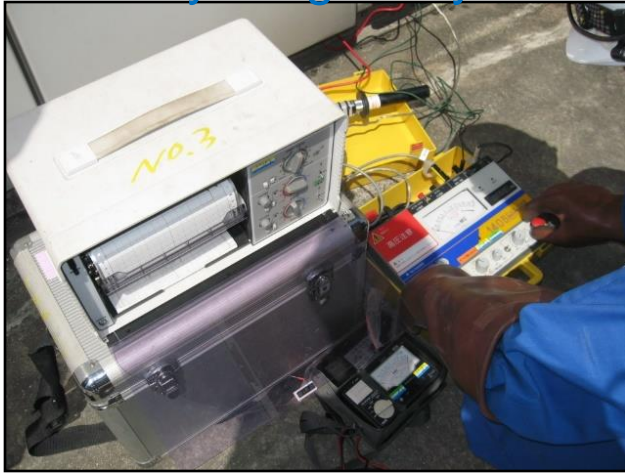
[Precision inspection of a high voltage CV cable]
