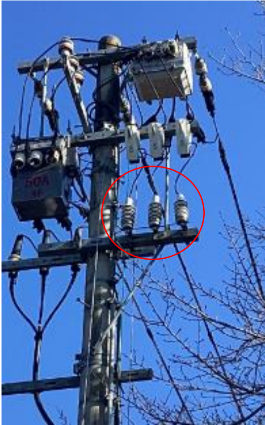
[Installation of a lightning arrester in a high voltage circuit]
