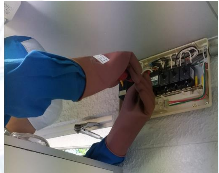
[Retightening of circuit breaker connections]
