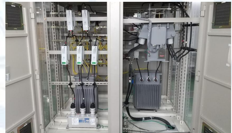
[Demand equipment of the cubicle type (back)]
